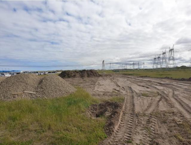
Image 8: Stockpiling of aggregate material.
