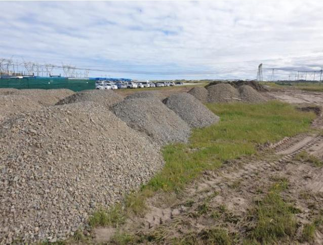
Image 7: Stockpiling of aggregate material.
